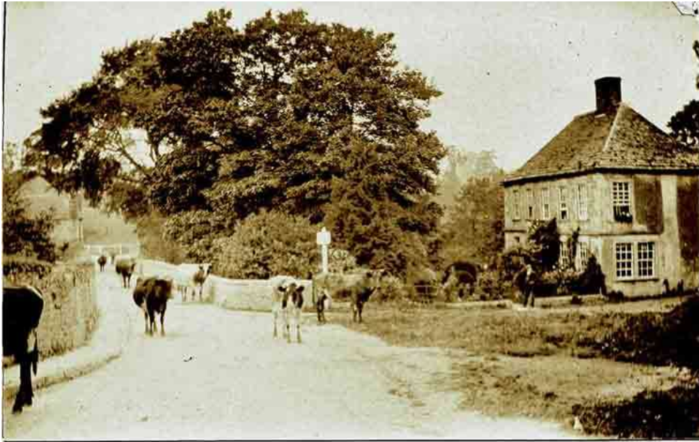
Figure 6 The Millers House and bridge c1900.
