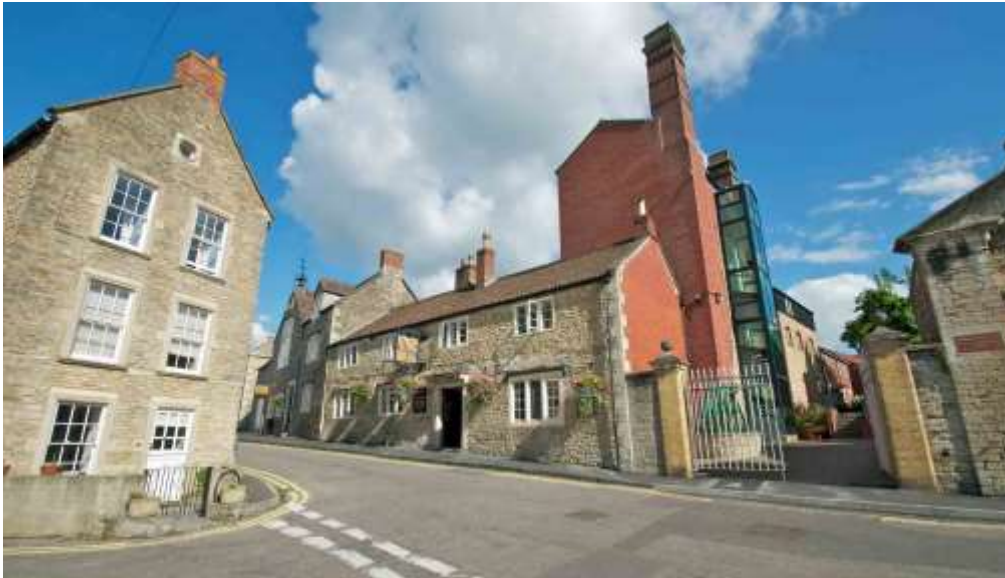
Figure 3 The Cross Keys Public House with the old Brewhouse now converted into apartments.
