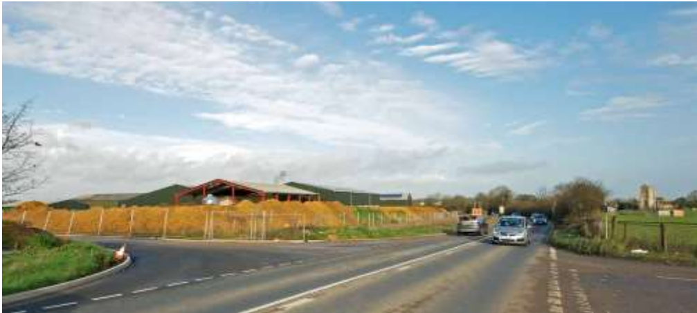
Figure 22 The Fussell development to the south of Rode nearing completion
